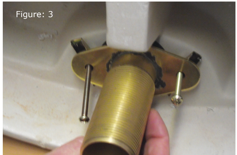
Figure 3: Using fixing bolts and butterfly clips screw waste fixing to basin.
