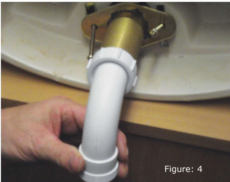
Figure 4: Fasten waste connector on to waste outlet.
