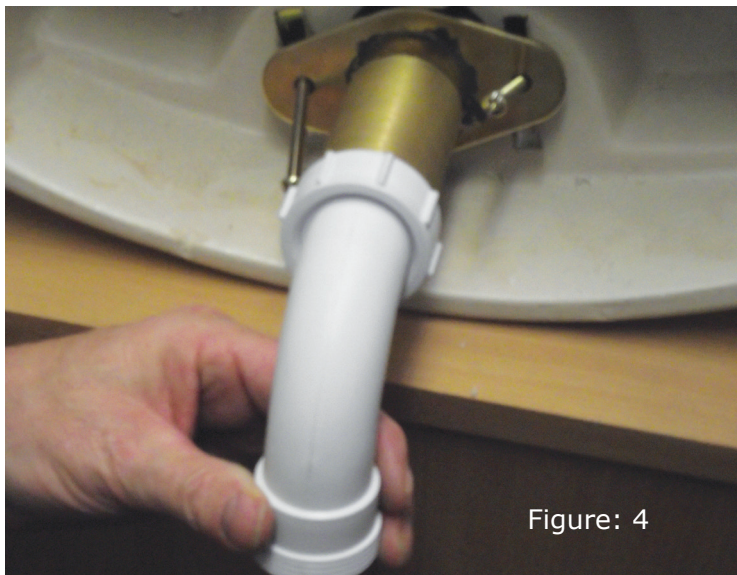
Figure 4: Fasten waste connector on to waste outlet.
